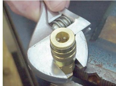
With even and smooth force applied, wrench tighten according to the 'Turns From Finger Tight' (T.F.F.T.) values listed below. DO NOT OVERTIGHTEN!
